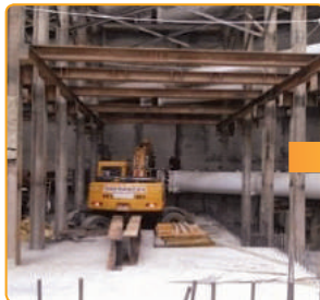
▲ Construction of Building SLAB in the Basement
