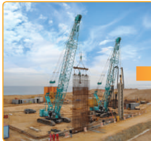
▲ Earth Retaining Wall Construction
