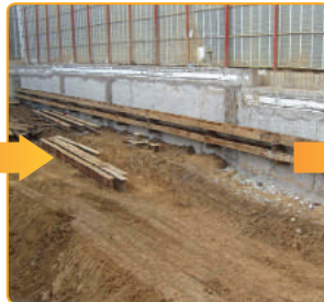
▲ Installation of Wale and Backfill
