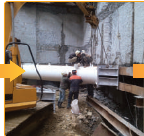
▲ PPS Installation (Placing of PPS and Connection)
