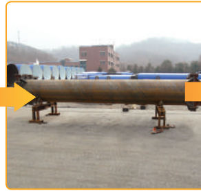
▲ Installation of PLATE of the End Part of Steel Pipe
