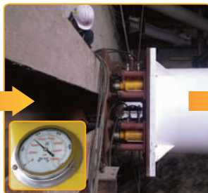
▲ Removal of Pressure from Prestressed Load Jack
