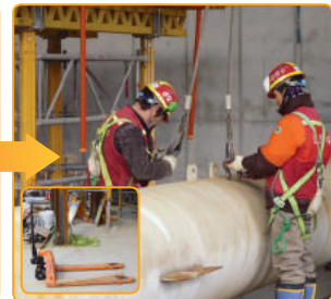
▲ PPS Dismantling (Transportation and Salvage)
