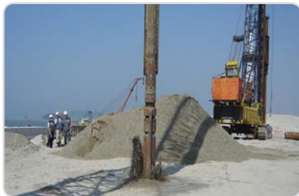
Probe Penetration stage within the ground
