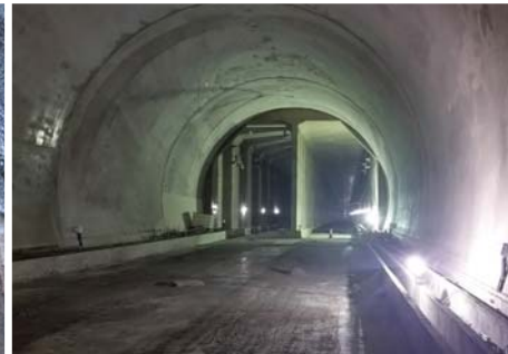
▲ The construction works of the Metropolitan Express Railway of Suseo-Pyeongtak (Section No. 1-2), Seoul
