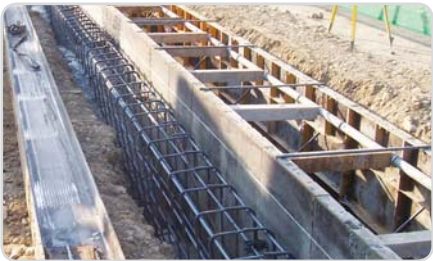
Placing of Steel Reinforcement
