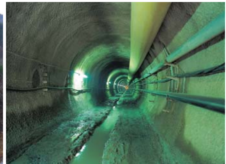
Metropolitan Double Line Construction for Tap Water, Seoul
