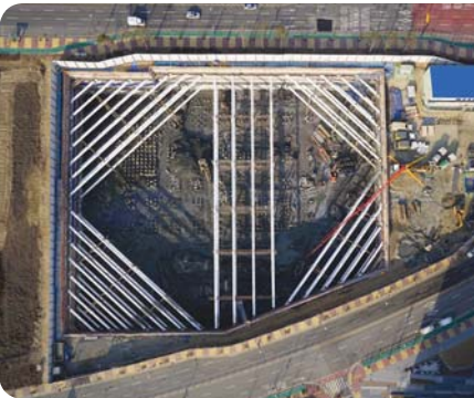
EBS Digital Integration Company office Building, Ilsan · Excavation depth : 13~16m · PPS installation layer & length : 2 layer / 2,356m · PPS diameter : Ø 800mm
