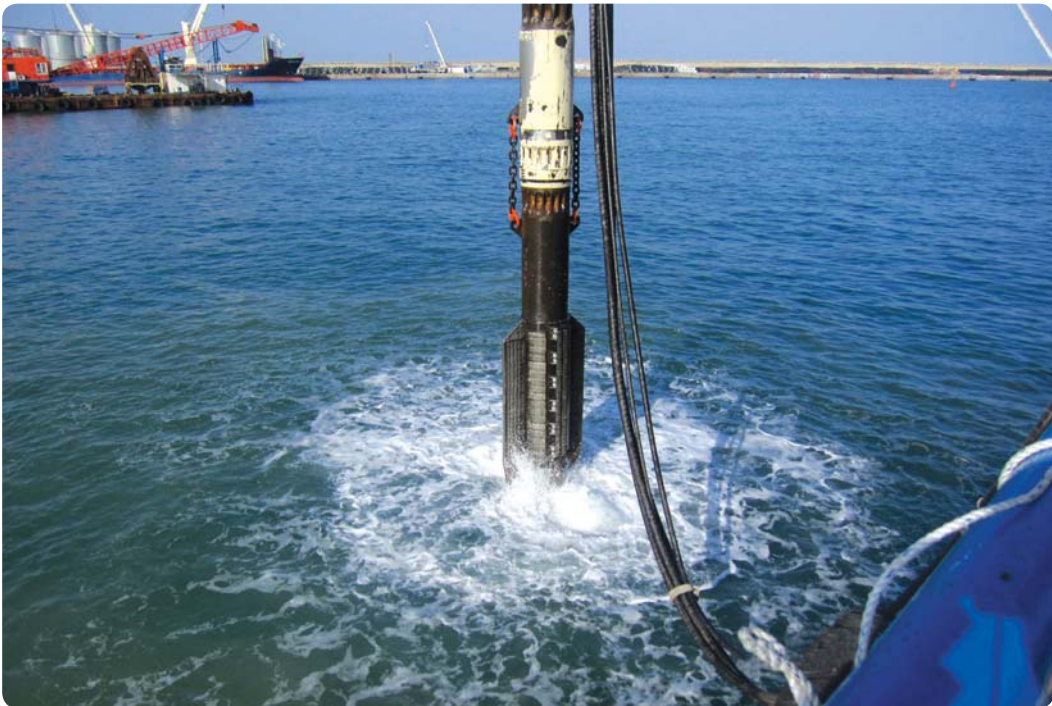
Construction of Stone Column for Substructure of Dock at Gunsan Shipbuilding Yard
