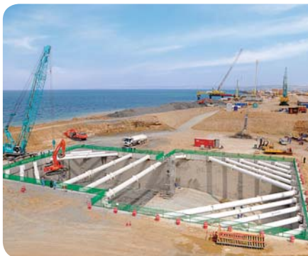
Algeria Oman Fertilizer Plant Intake (ALGERIA) · Excavation depth : 10m · PPS diameter : Ø 800mm / Ø 1,000mm
