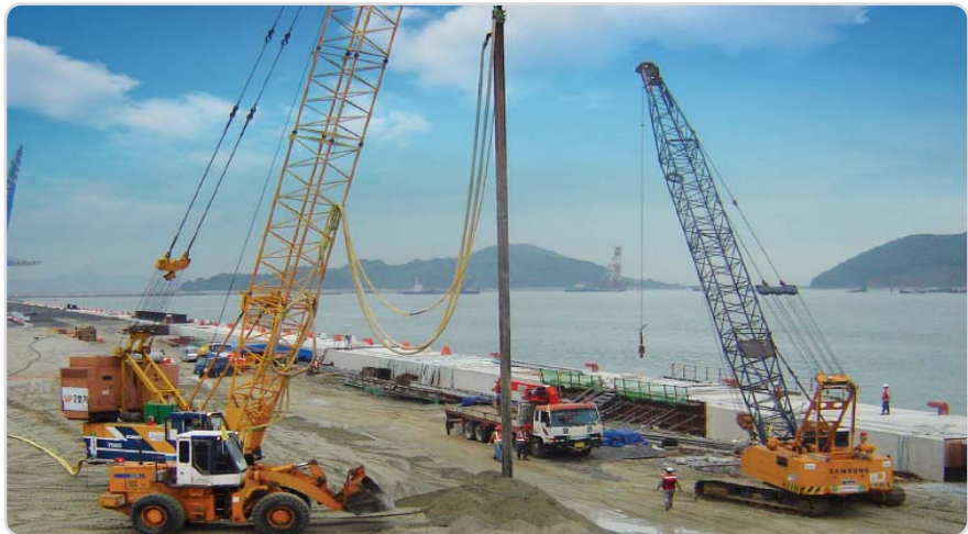
Busan Newport Phase 1-2, Vibro compaction site view
