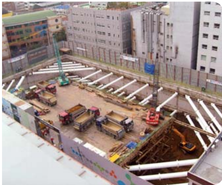
Sungsu Wooribank Call center · Excavation depth : 17.5~21.0m · PPS installation layer & length : 2~3 layer / 1,400m · PPS diameter : Ø 800mm
