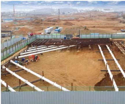
Wirye New City IS Central Tower · Excavation depth : 14.0~18.5m · PPS installation layer & length : 3~4 layer / 1,740m · PPS diameter : Ø 800mm
