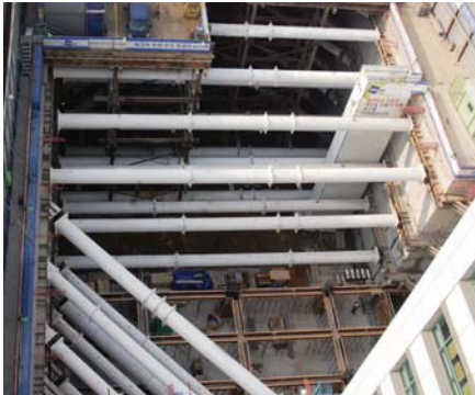
Sangam Doosan Weve Centium, Seoul · Excavation depth : 19.0~23.0m · PPS installation layer & length : 3~4 layer / 840m · PPS diameter : Ø 800~1,000mm
