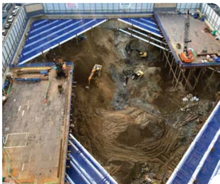
Pyungchon IS BIZ tower, Anyang · Excavation depth : 16.3~19.3m · PPS installation layer & length : 3 layer / 2,707m · PPS diameter : Ø 800mm
