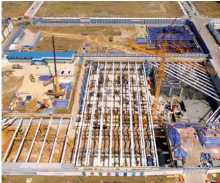
Magok Kolon the Future technology center · Excavation depth : 13.9~17.9m · PPS installation layer & length : 2 layer / 3,260m · PPS diameter : Ø 800mm
