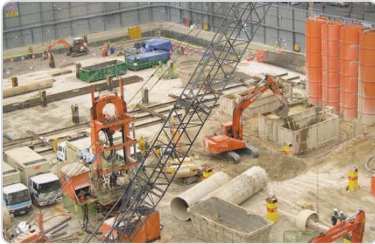
RCD construction scene at Good Morning City
