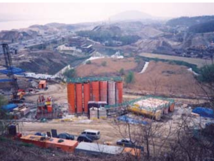
Nanjido Cut-off Wall, Seoul
