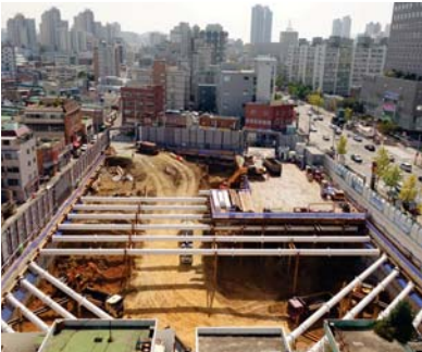
▲ Gwangsan Mansion Reconstruction Project, Busan
