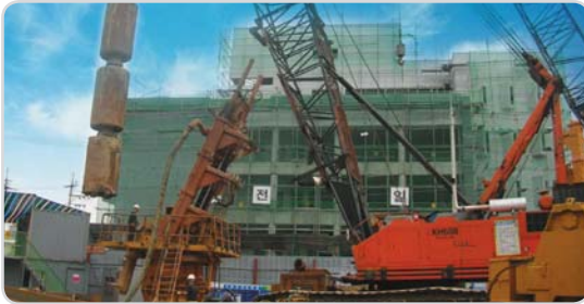
RCD construction at Hanil Residential Complex Building in Mangwoo-dong
