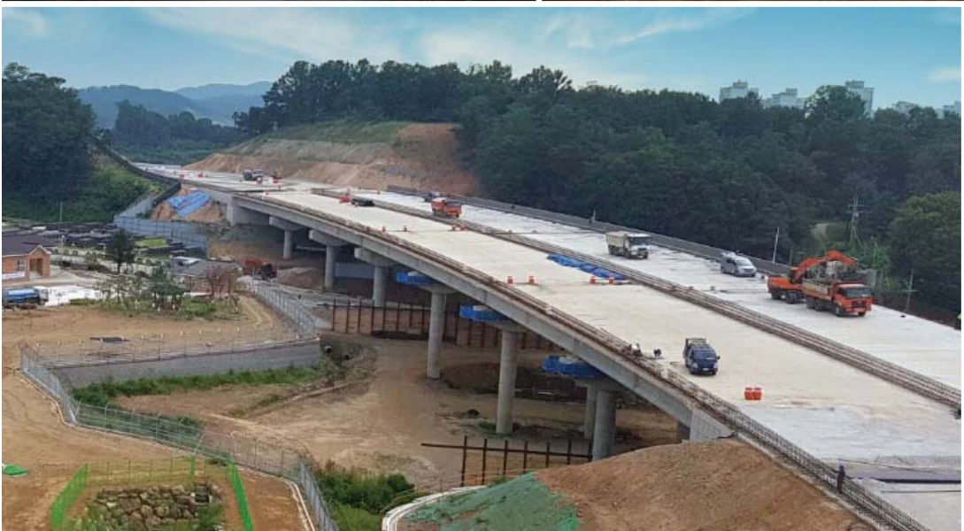
▲ The construction works of the Highway of Guri-Pocheon (Section No. 3), Namyangju
