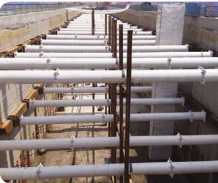
Incheon Airport Second Passenger Terminal, Incheon · Excavation depth : 21.0~25.0m · PPS installation layer & length : 2~3 layer / 6,000m · PPS diameter : Ø 800mm
