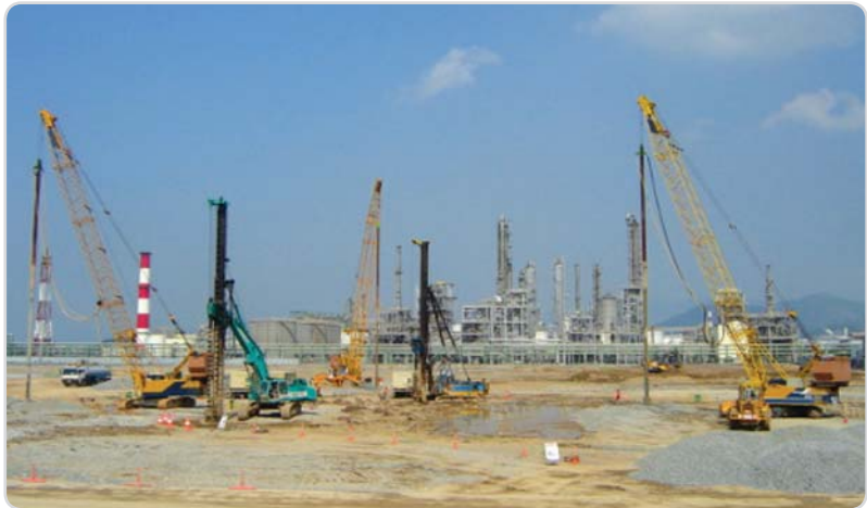
HOU No.2, VDU Tank Area GS CALTEX, Yeosu
