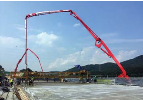
▲ The construction works of the Highway of Guri-Pocheon (Section No. 3), Namyangju
