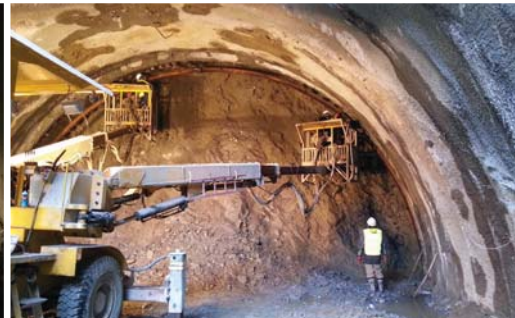
▲ The construction works of the Metropolitan Express Railway of Suseo-Pyeongtak (Section No. 1-2), Seoul
