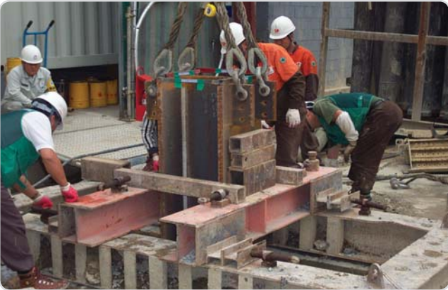
Installation of Barrette Steel Frame
