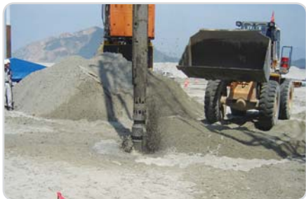
Drawing and compaction steps
