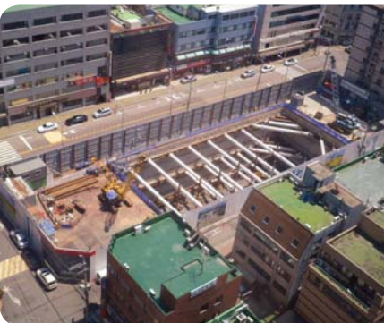
Jamsil I-Park Officetel, Seoul · Excavation depth : 18.8~23.7m · PPS installation layer & length : 3 layer / 1,000m · PPS diameter : Ø 800mm
