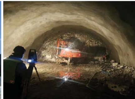
▲ The construction works of the Highway of Guri-Pocheon (Section No. 3), Namyangju
