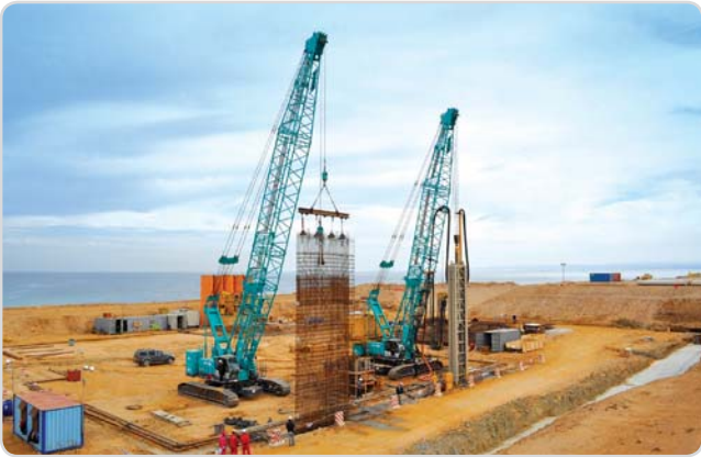
Placing of Steel Reinforcement
