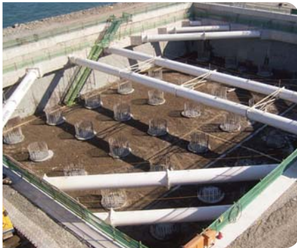
North Port Bridge Marine Special Foundation, Busan · PPS installation layer & length : 1 layer / 250m · PPS diameter : Ø 1,200mm
