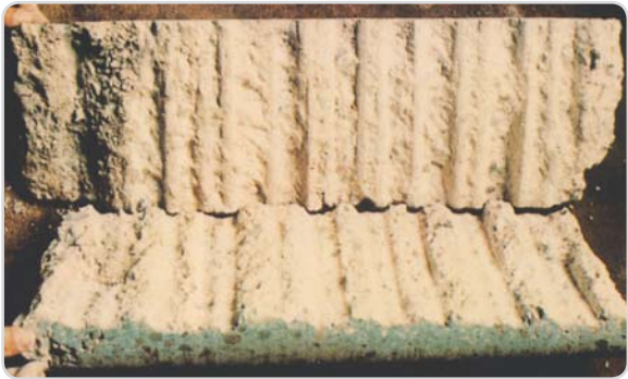
Detail View of Joint
