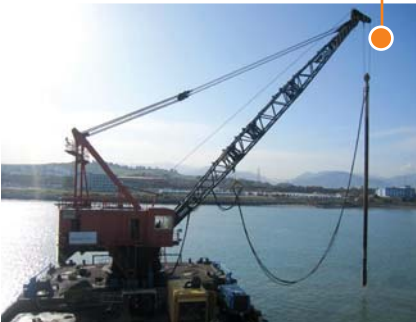
▲ Algeria Djen Djen Port, harbor structure extension work (ALGERIA)
