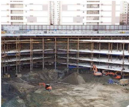
Yonghoman Complex Facility, Busan · Excavation depth : 21.5m · PPS installation layer & length : 4 layer / 1,850m · PPS diameter : Ø 800mm
