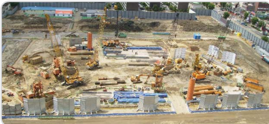
RCD construction scene at Poonglim Exllu Tower in Incheon
