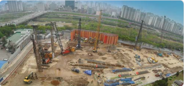
Barrette Pile Construction Scene at National Assembly Member's Office Bldg. in Yeouido
