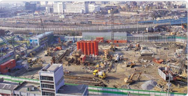
Barrette Pile Construction Scene at Byeoksan Mixed-use Apartment in Hangang-ro
