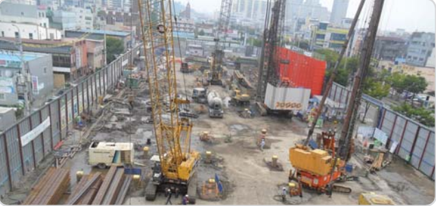
Barrette Pile Construction Scene at Upsquare in Ulsan
