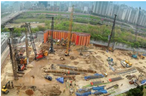
National Assembly Member's Office Bldg., Seoul
