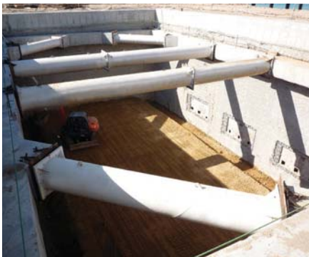
Algeria Oman Fertilizer Plant Outfall (ALGERIA) · Excavation depth : 11.9m · PPS diameter : Ø 800mm / Ø 1,000mm
