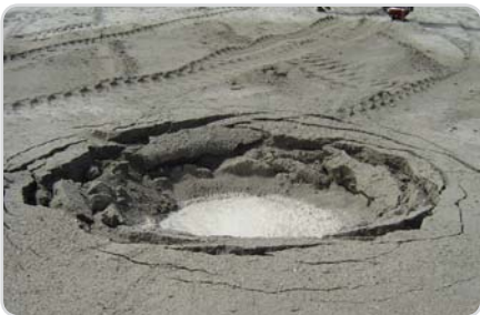
After Completion Vibro Compaction
