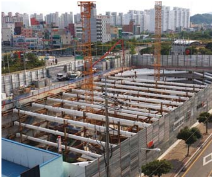
Kwangyang E-Pyeonhansesang APT · Excavation depth : 15.5~20.9m · PPS installation layer & length : 3 layer / 2,320m · PPS diameter : Ø 800mm
