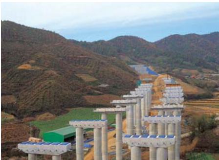
Jungbu Naeryuk Expressway, Mehyun bridge work, Chungju
