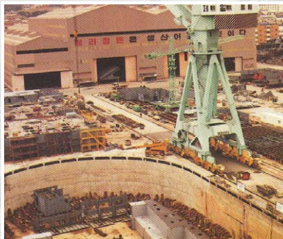
거제상선조선소 Dry Dock
