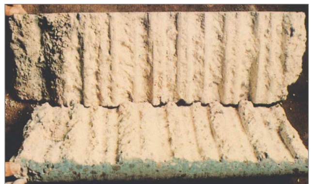
Deail View of Joint
