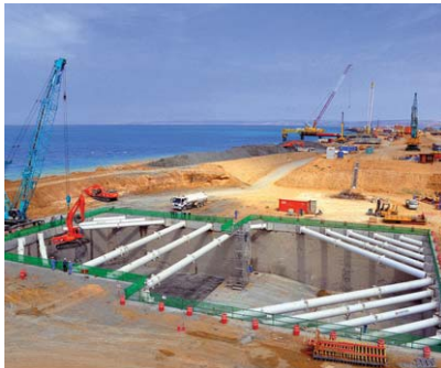
Algeria AOFP Project (Intake Basin)
