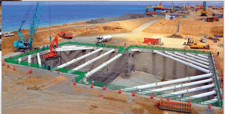
Algeria AOF Project(Intake Basin)
